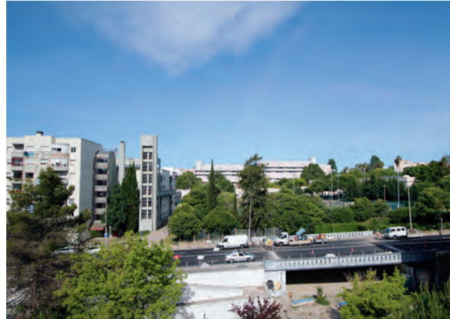
Fig. 4: Underpass pathway, photo 2021
