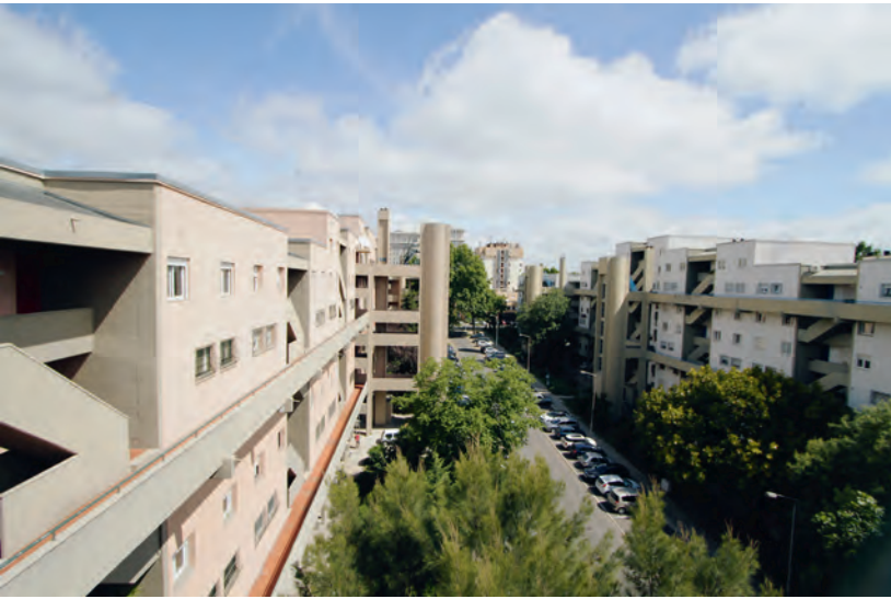
Fig. 2: Building block with exterior galleries, photo 2021
